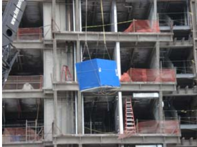
Air Handler Hoisting
