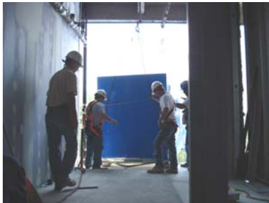
Rigging into the Mechanical Room
